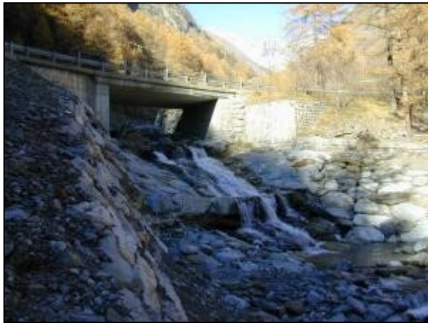
Opere anti erosione – Erosion Control
