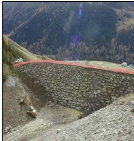
Opere paravalanghe / avalanche protection works
